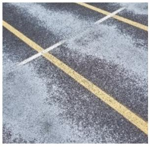
Current track is at end of life—sinkhole, worn surface, cuts in the track
