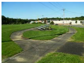
Asphalt paths and bleacher pad at AHS baseball field
